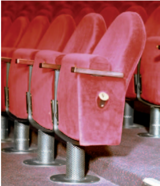
Figure 3: Seat displacement outlet, photograph
